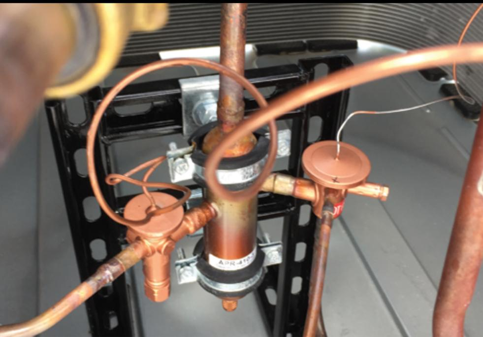
**A field-installed APR Control (by Rawal Devices) for variable capacity modulation on a 5-ton R-410A roof-mounted package unit. Image courtesy of Rawal Devices Inc.**
