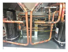
Since its introduction, the APR Control has been referred to as a continuous capacity modulation device based on the theory of modulating the adiabatic process of a refrigeration system. The APR was an unprecedented offering with no equivalent in the market. As APR Control was embraced by the industry, the most common and comparable reference was hot gas bypass.
